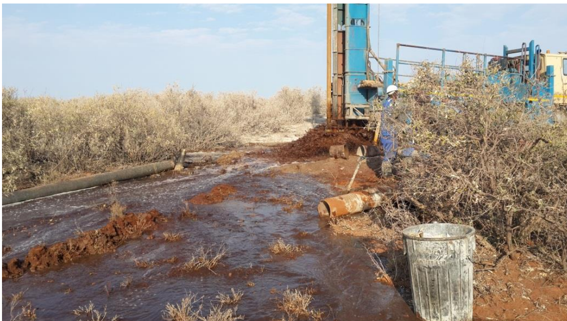
Figure 24: Drilling of SD2 -11
