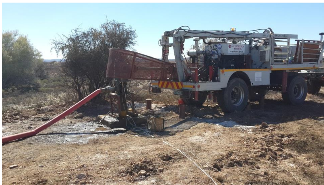
Figure 32: Aquifer Testing SD2-3
