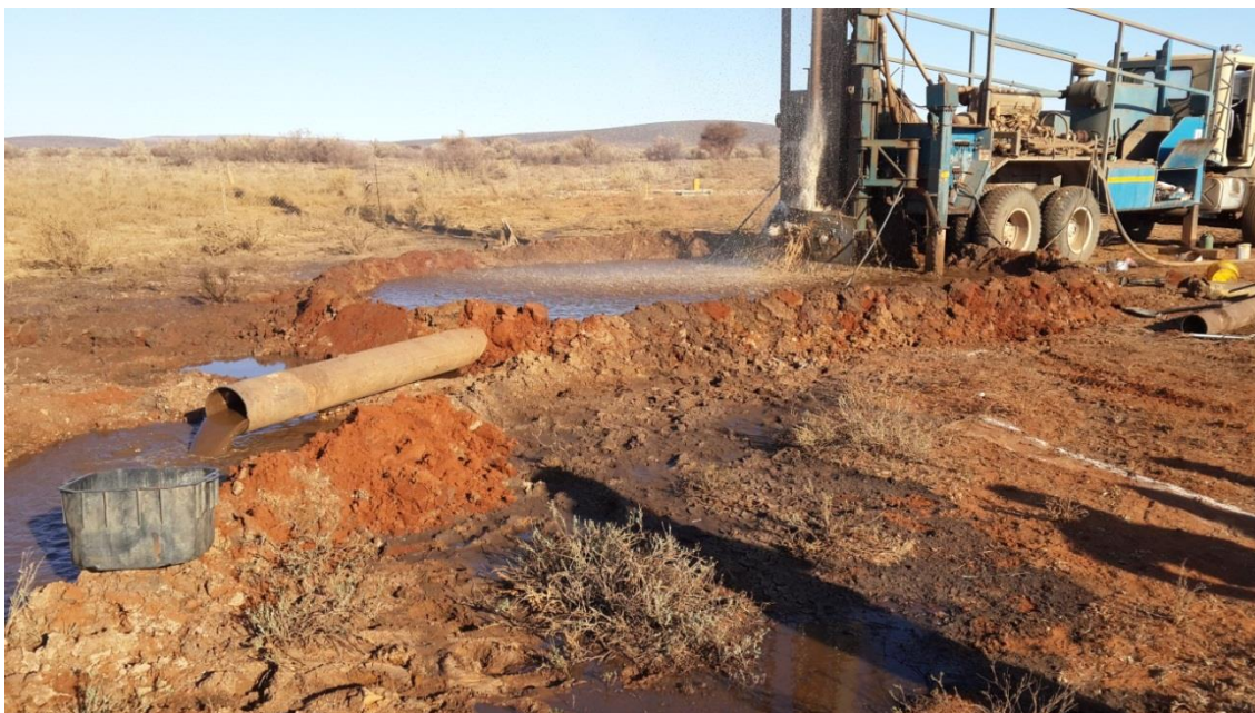
Figure 22: Drilling of SD2-16 with SD2-16M in Background.
