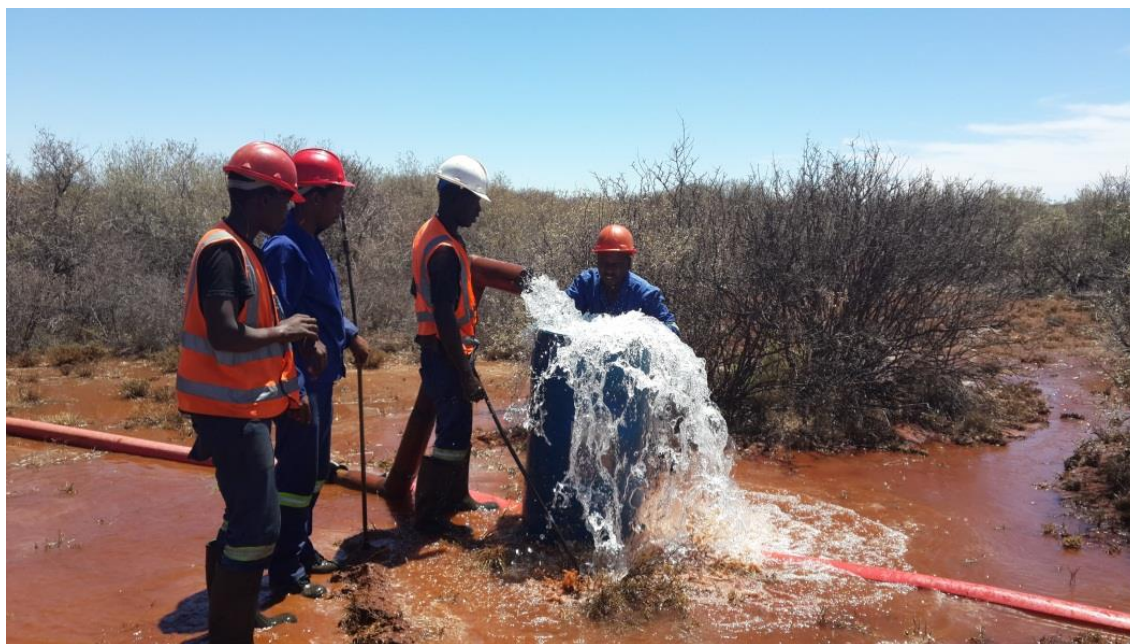
Figure 33: Aquifer Testing of SD2-26 (20l/s)
