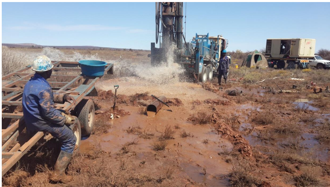
Figure 20: Air Percussion Drilling Rig - SD2-09
