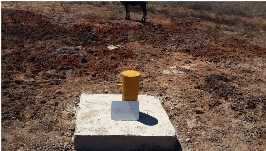
Figure 25: SD2-16 Completed Headwork's
