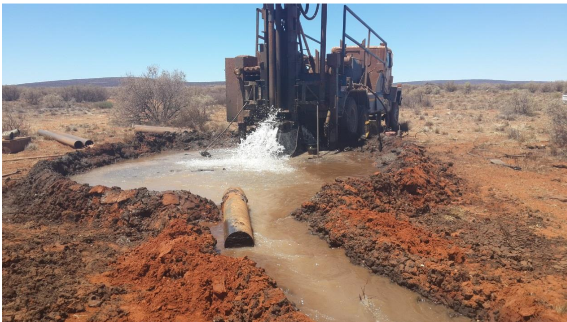
Figure 21: Drilling of SD2-30- BY 30.0 l/s
